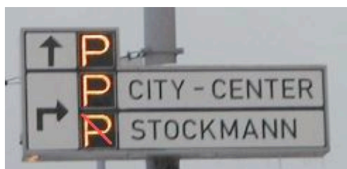
Figure 5. Variable message signs for parking as part of the HelUTC system.
